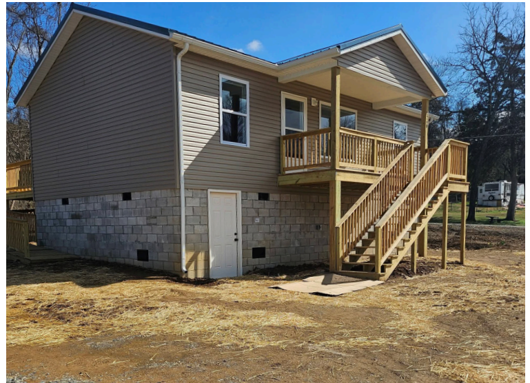
New home construction underway
